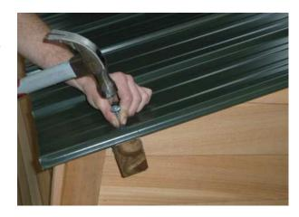
Step 17: Lay out remaining full roof sheets and 1/2 sheet. Rivet these sheets together, 2 rivets per join, to make 1 large roof panel as shown in photo. Tack remaining top corner and bottom corner ensuring edge of sheet is flush with end of purlins and height is correct.
